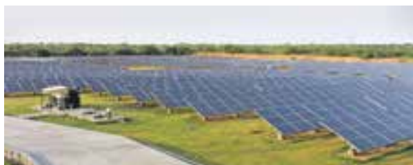
GTPS Ash Dyke, 1MW SPV Power Plant, Gandhinagar
