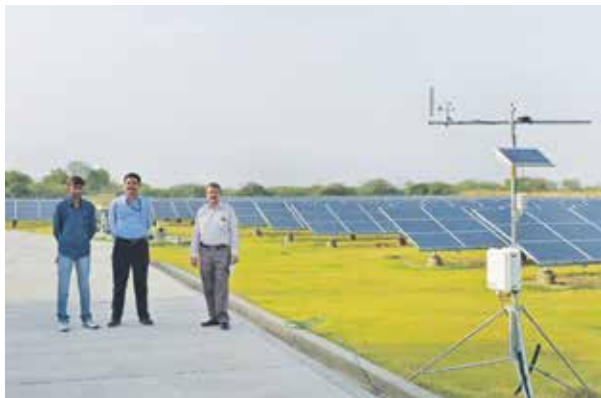
IRADe research team on visit to 1 MW solar power plant on Ash Dyke of the 850 MW Gandhi Nagar thermal power station, Gandhi Nagar
